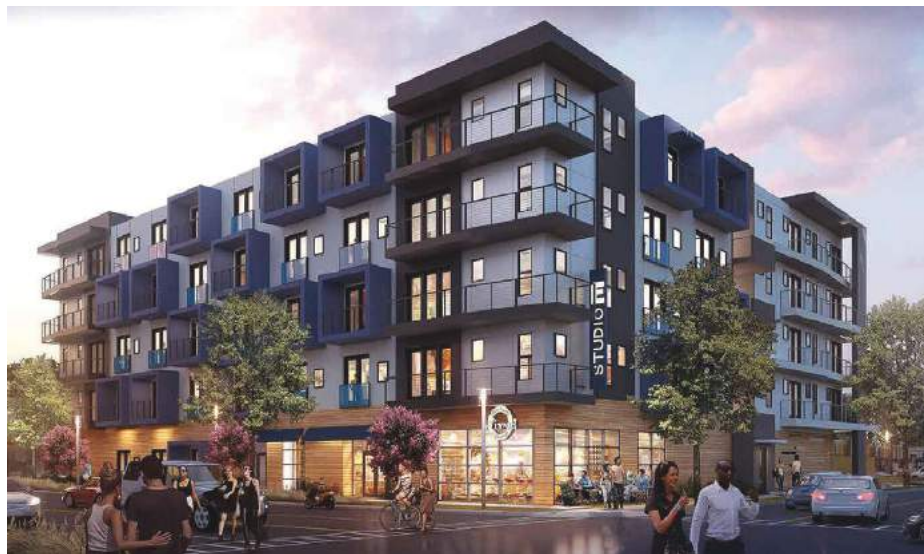
Transwestern Development is underway on the 139-unit Indie Apartments, a micro-unit community in East Sixth, an entertainment district just east of downtown Austin.
